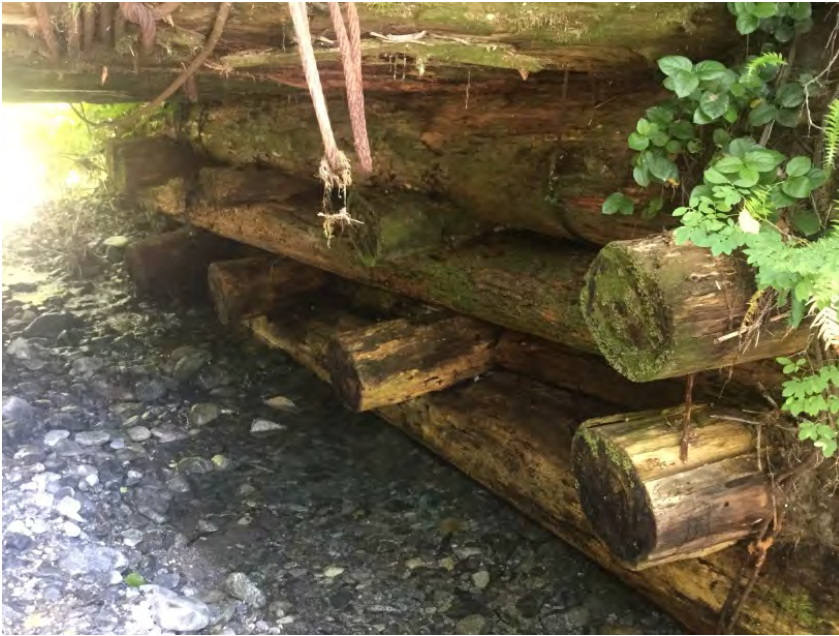
Left Bank Abutment
