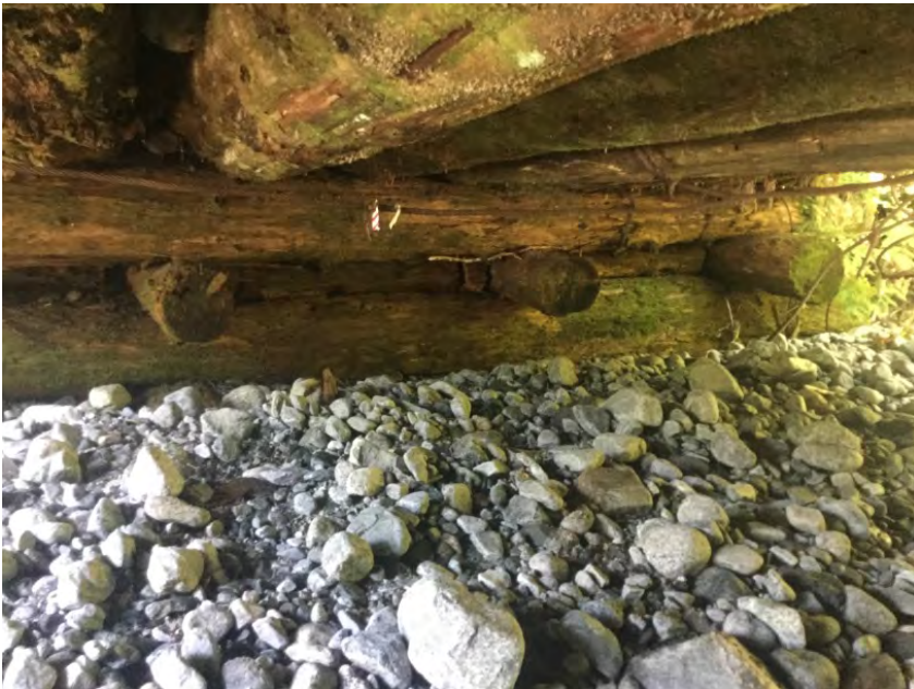
Right Bank Abutment
