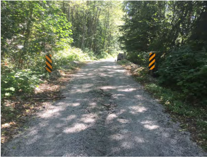
Right Approach Facing Bridge
